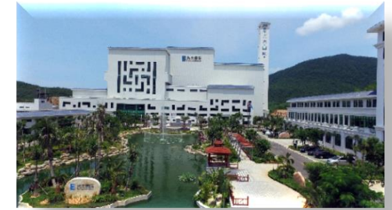
Hainan Sanya Waste-to-energy Project
