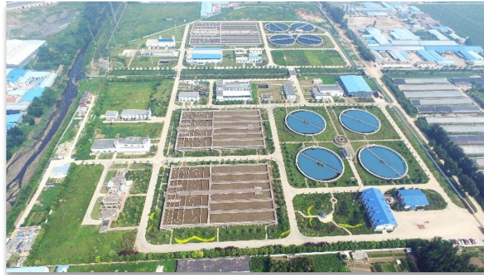
Ji'nan No. 3 Waste Water Treatment Plant
