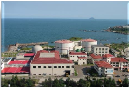
Qingdao Waste Water Treatment Project
