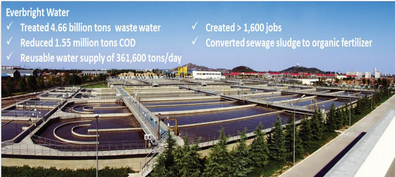
Ji'nan No. 2 Waste Water Treatment Plant
