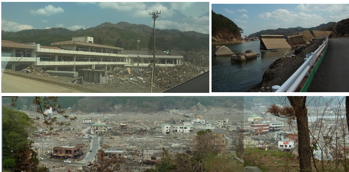
A middle school in Kamaishi: flooded to the third floor (top left), A levee destroyed by tsunami (top right), Otsuchi town totally devastated (below)
